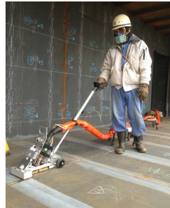
An ENRX Terac system ensures failsafe operation – it makes it impossible to overheat magnetic steel. Moreover, Terac does not produce toxic gases from the heating source. And, there is no acoustic noise.
