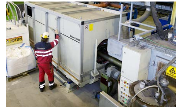
A medium-frequency ENRX Sinac pre-heats seamless offshore pipe prior to coating.
